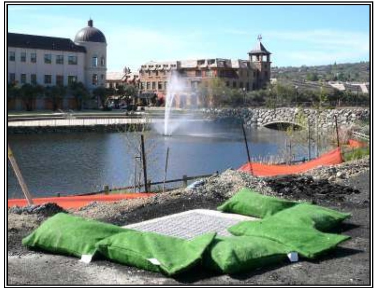
The Heavyweight™ Bags newly installed.
