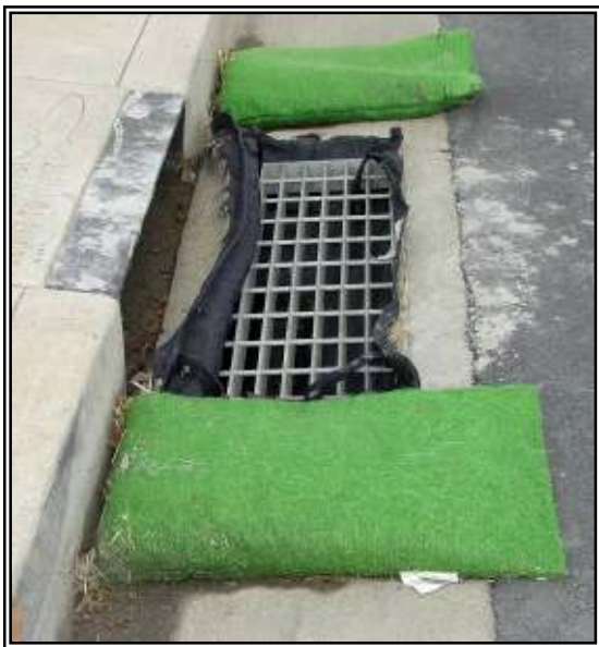
The Heavyweight™ Bags installed around drain inlet, six months later.
